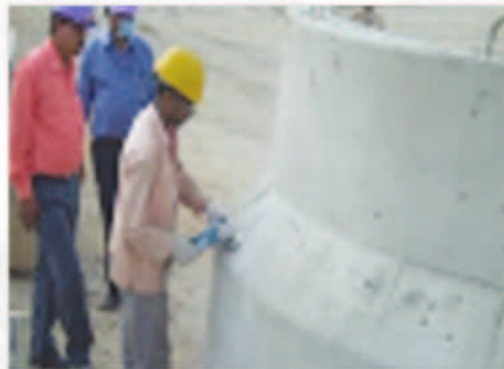
Grinding Preconcrete
