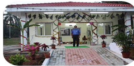
New Block for Security Office
