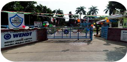
Entrance to the factory
